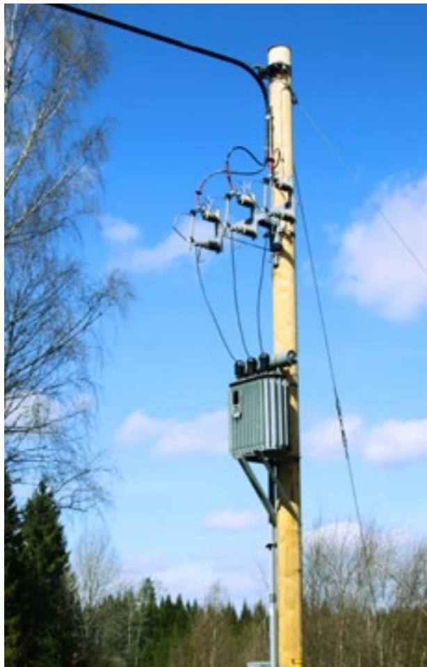
Pole-mounted substation.
