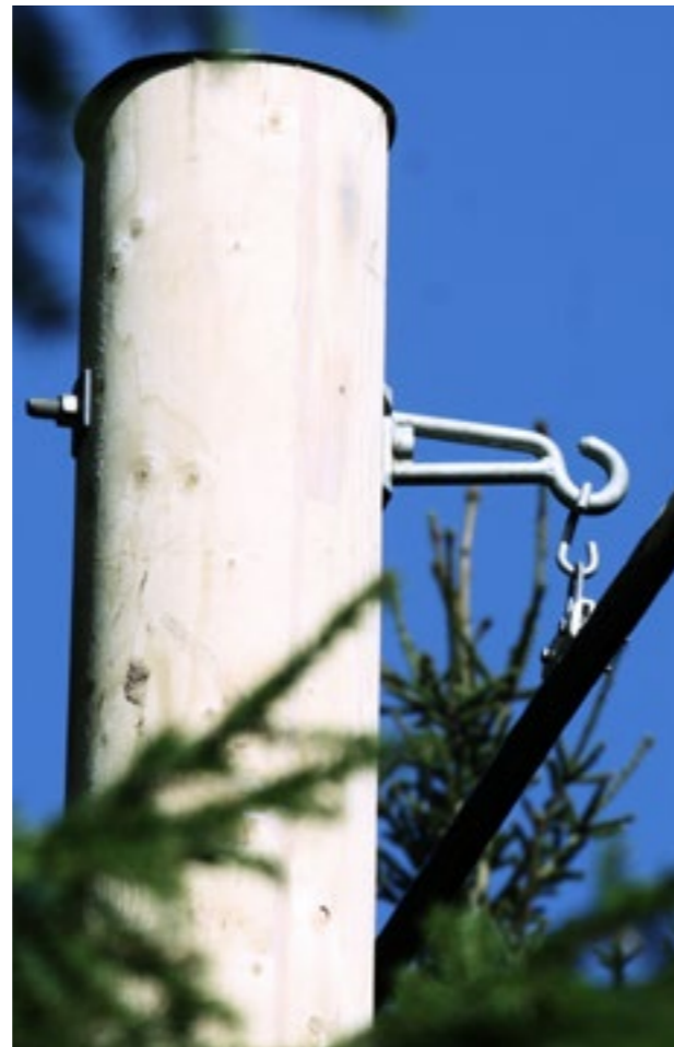
Suspension with breaking link.
