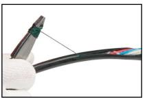
Remove the sheath and cut off all the yarns and tapes lying around the fiber tubes. Wrap off the fiber tubes from the reinforcing member (FRP) and cut off FRP in an appropriate length.
